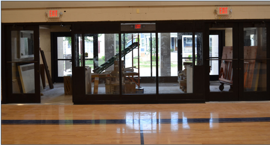
New Interior Doors (Gym Entrance)
