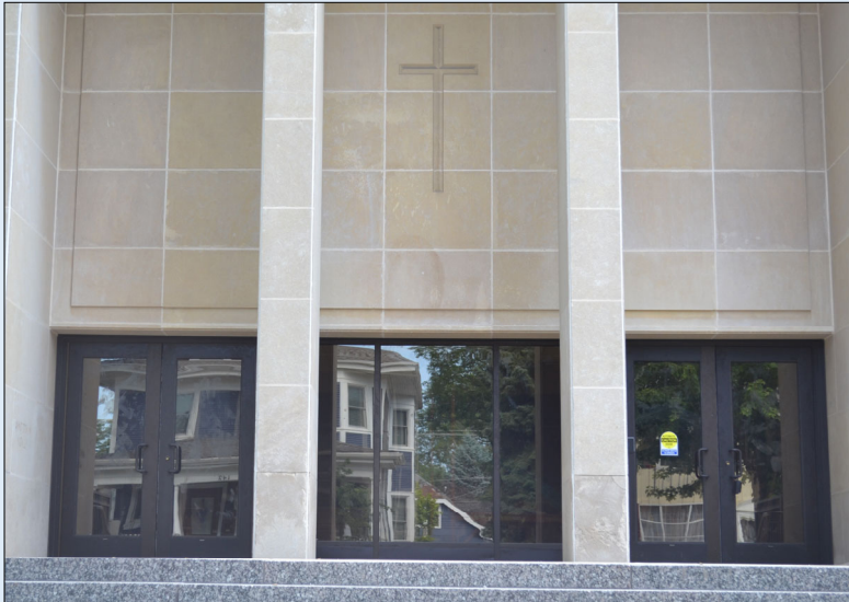
New Exterior Doors (Gym Entrance)
