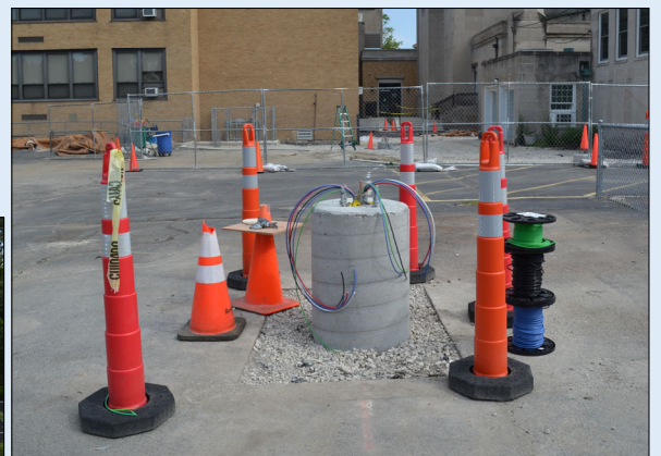
New Electrical for Light Posts
